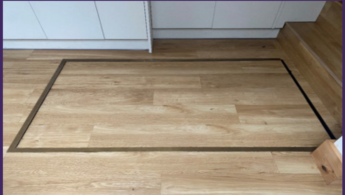
Invisible Step Lift by Oyster Mayfair now concealed in pit.
