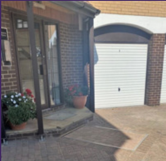
Lift at rest concealed under to paving.
