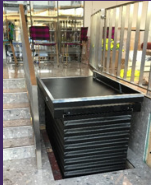
A model V (for vertical travel only) being installed in a restaurant.
